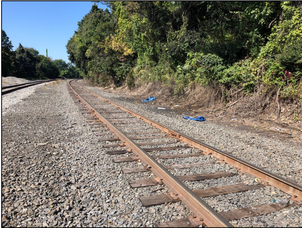
View of Dover & Delaware Eastbound main track, facing west. New Westbound main shall be constructed between Eastbound main and embankment on existing subgrade.
